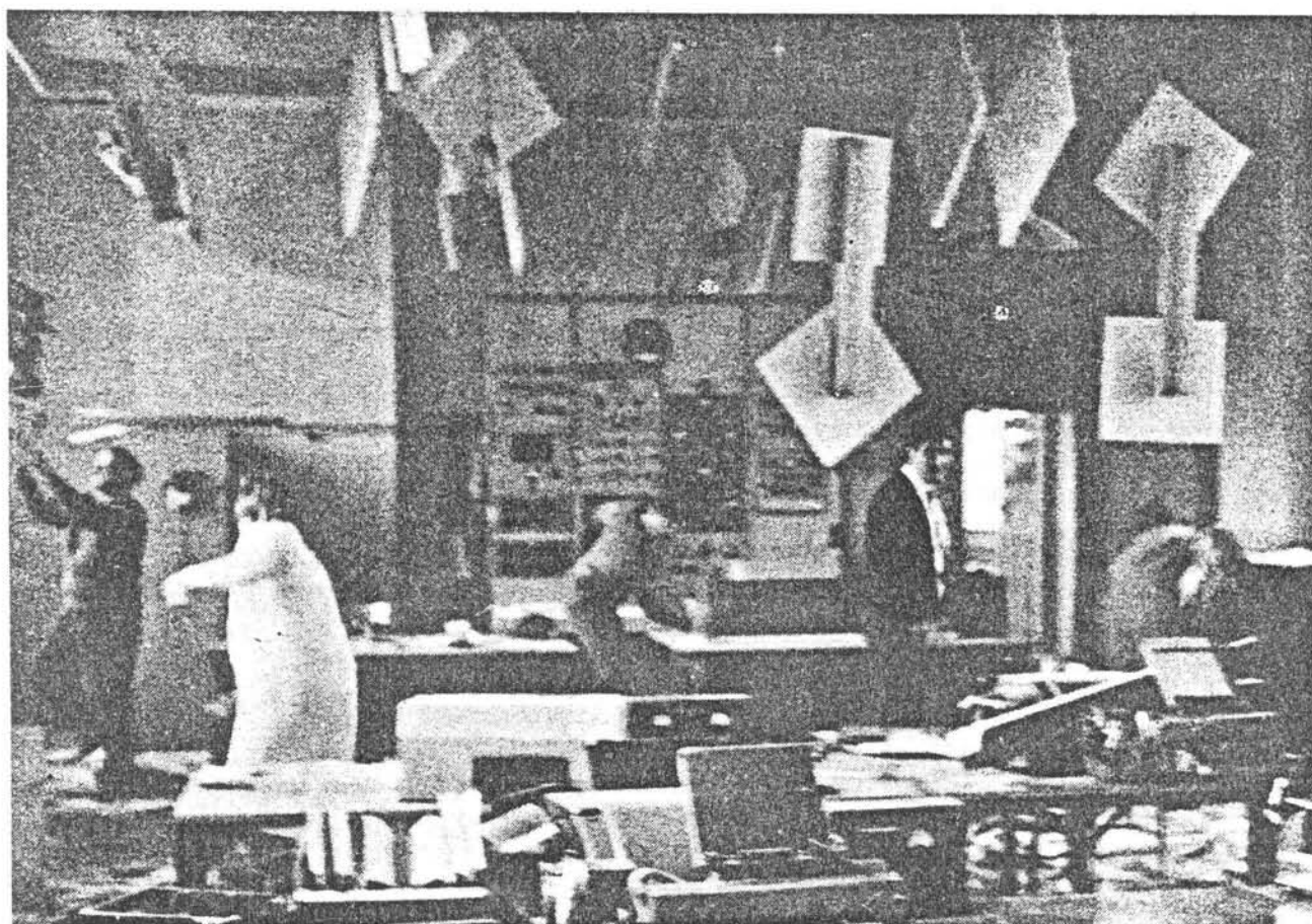
Interior of Greymouth Telegraph Office showing damage to ceiling tiles (NZ Society for Earthquake Engineering, Bulletin , vol. 2, no. 1, 1969, p. 76).
