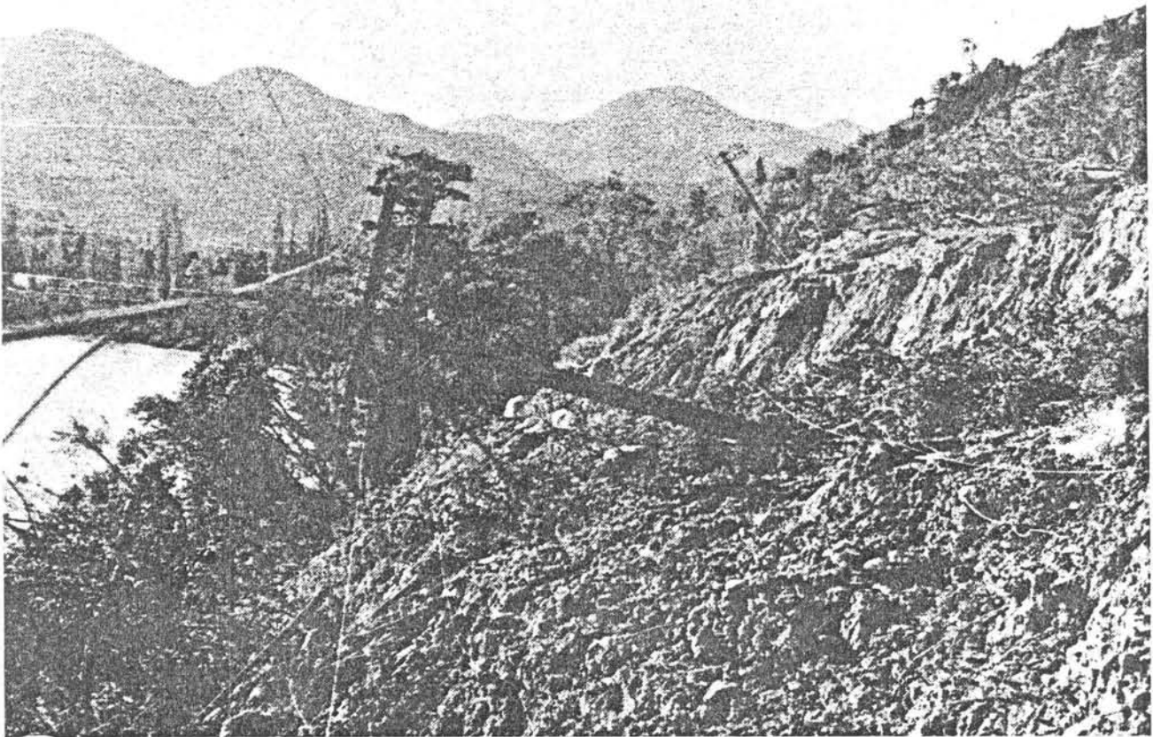
Typical damage to poles near New Creek, 12 km up the Buller Gorge from Inangahua Junction. Cut telephone lines hampered the Civil Defence response for some time (NZ Society for Earthquake Engineering, Bulletin , vol. 2, no. 1, 1969, p. 76).
