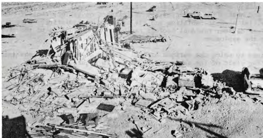
Effects of 5 psi overpressure
