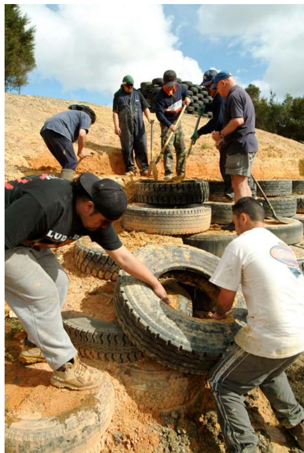
Community work being carried out.
