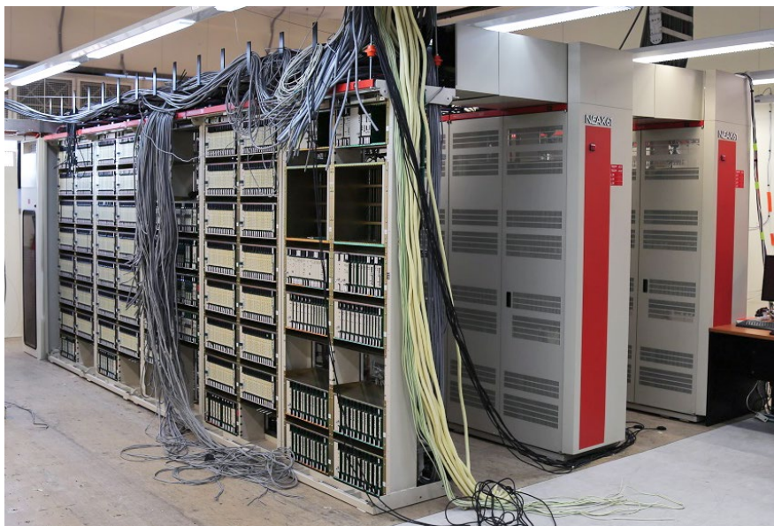
PSTN switches being decommissioned.
