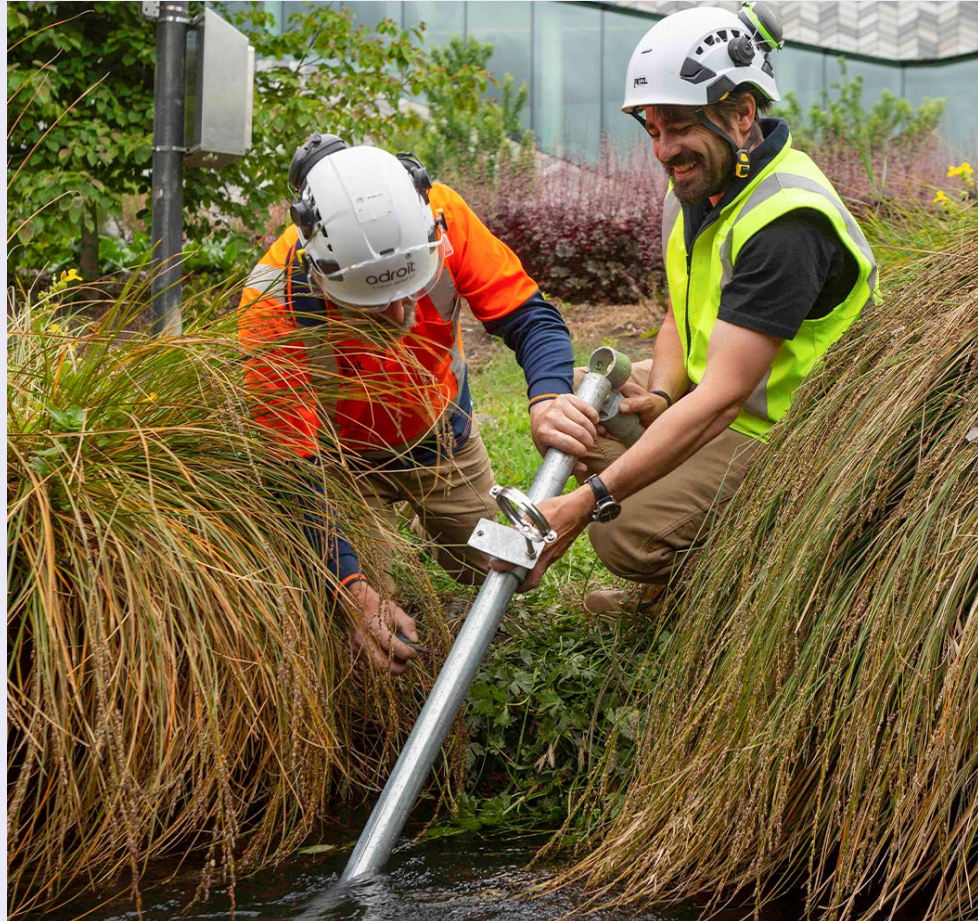
Water sensors have been installed near various water sources along the Ōtākaro-Avon river enabling Christchurch City Council to respond quicker to water contamination events.
