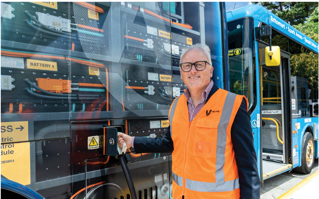
Launch of New Zealand's first fully electric bus depot with the capacity to charge 20 - 30 buses each. Charging at this depot occurs within a 'dynamic operating envelope', where Vector forecasts optimal charging times each day and provides this through to the depot, reducing peak demand for a more affordable charging solution.
