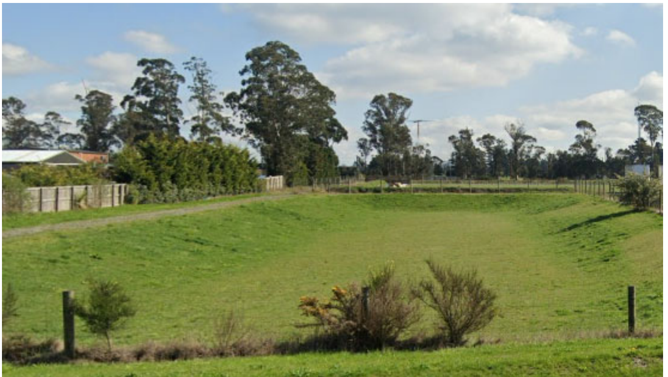
Figure 24 Typical Stormwater Basin – Example
